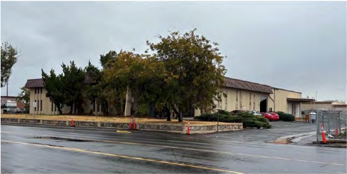
Old Textron Building Abatement in Progress
