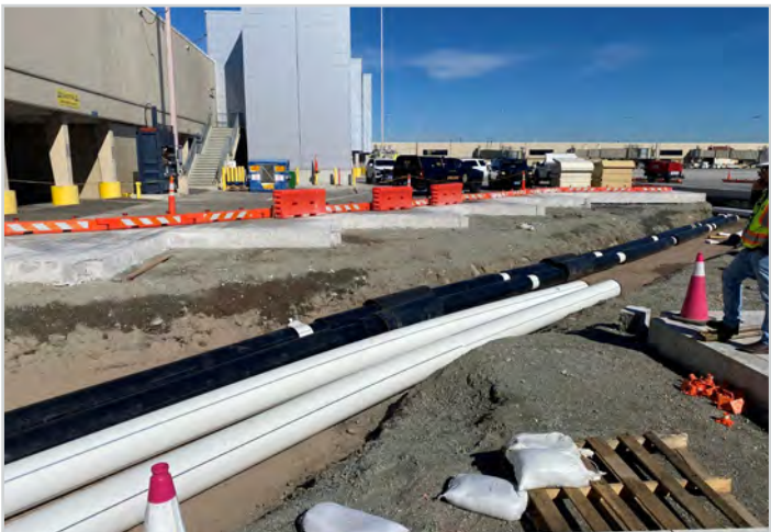
Trench - Phase 6c
