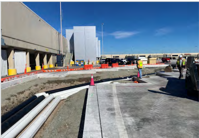
Trench - Phase 6c
