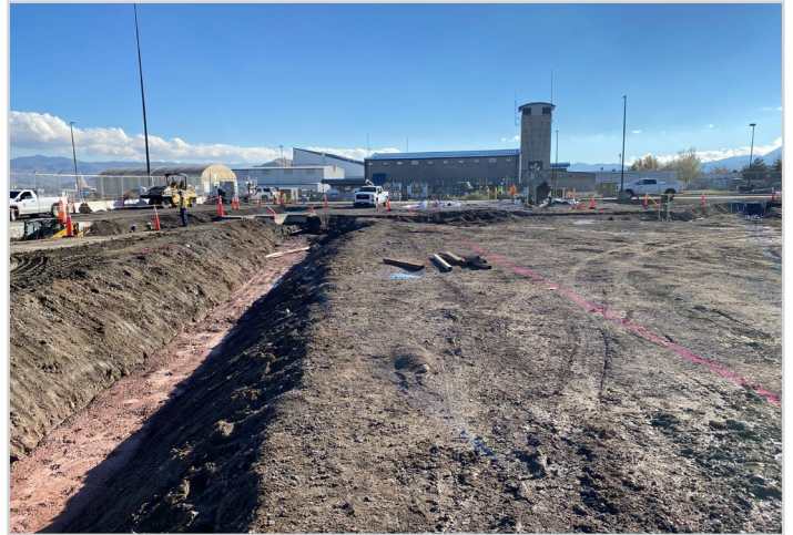
Utility Trench with Slurry
