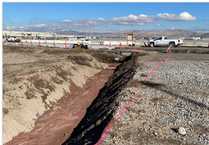
Utility Trench with Slurry
