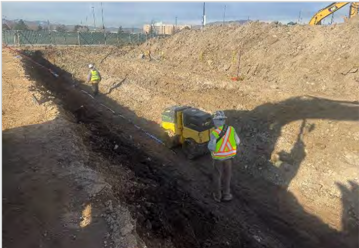
Compacting trench fill for fire line
