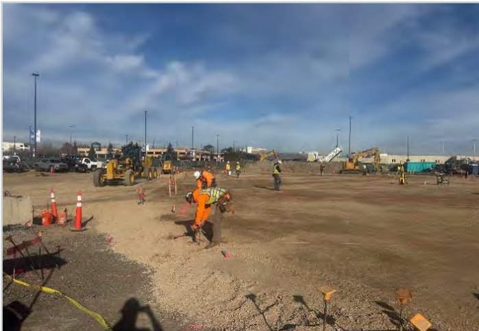
Setting batterboards for pad
