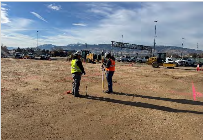
Verifying grade for MEP excavation
