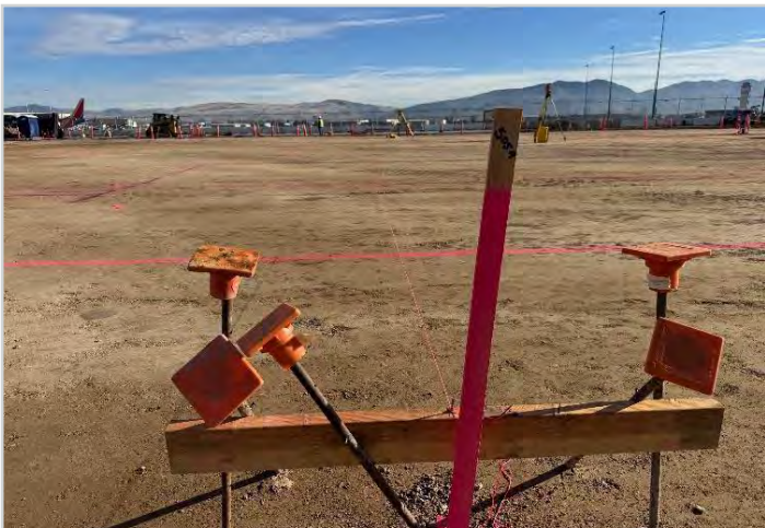
Batterboard set with string line
