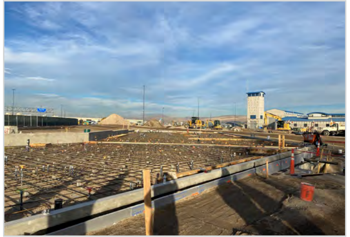
Building Slab on Grade Rebar
