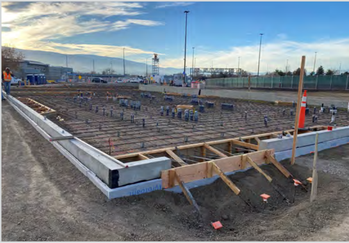
Building Slab on Grade Rebar
