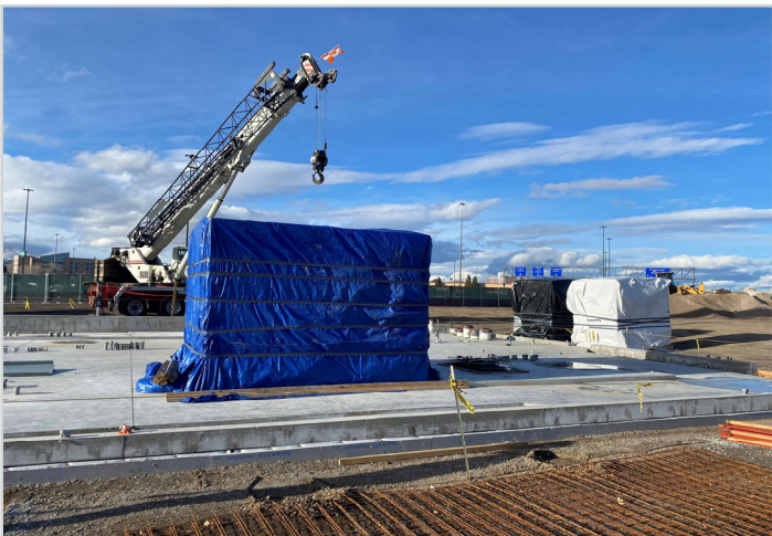
Setting electrical gear
