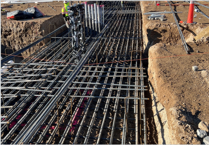
Utility conduit and rebar for footings
