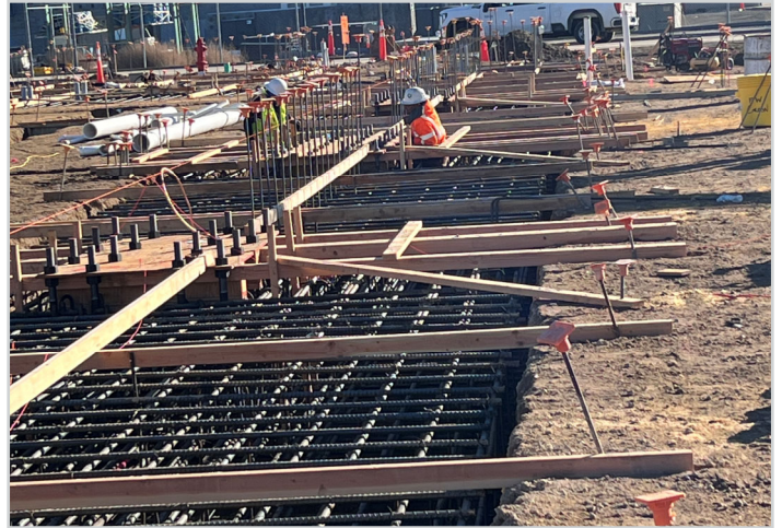
Installing rebar for footings
