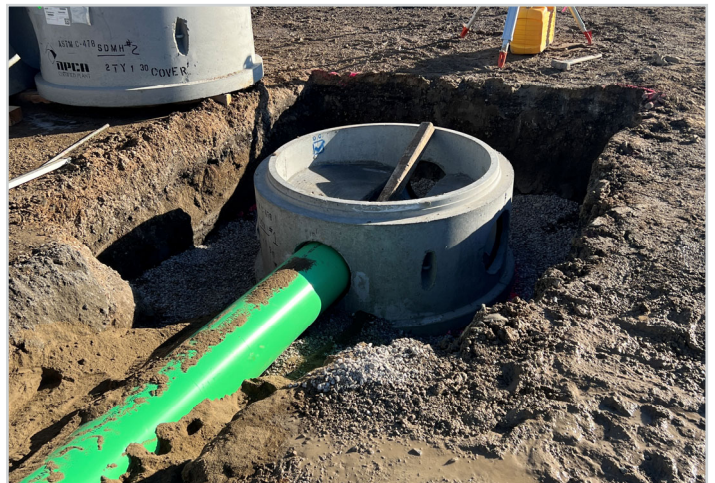
Installing storm drain manhole
