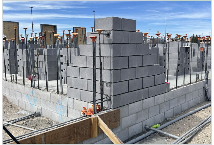
CMU Block Installation
