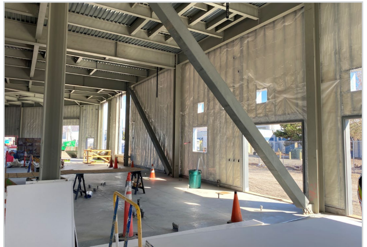
CUP Interior Insulation
