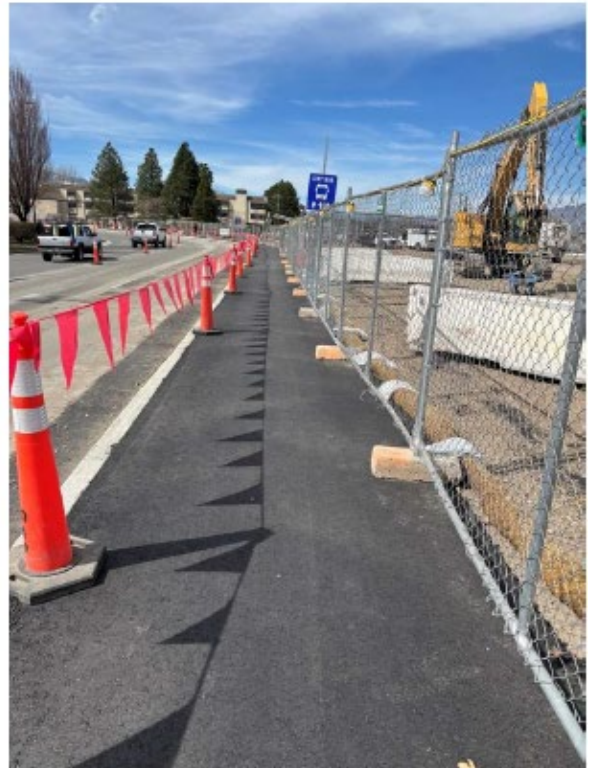
Temp Pedestrian Walkway
