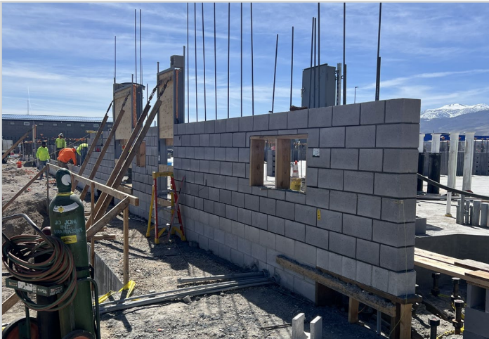
CMU Block Installation
