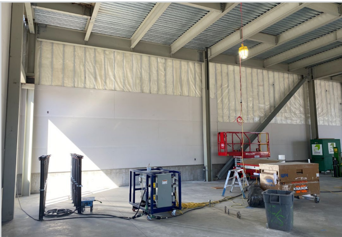
CUP Interior Drywall & Insulation
