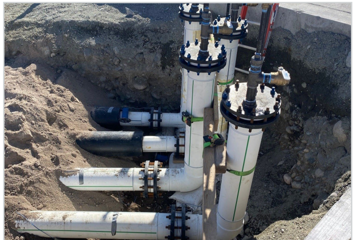
CUP Trench Area 7E - Hydraulic Piping
