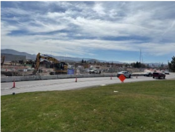
Terminal Way Work
