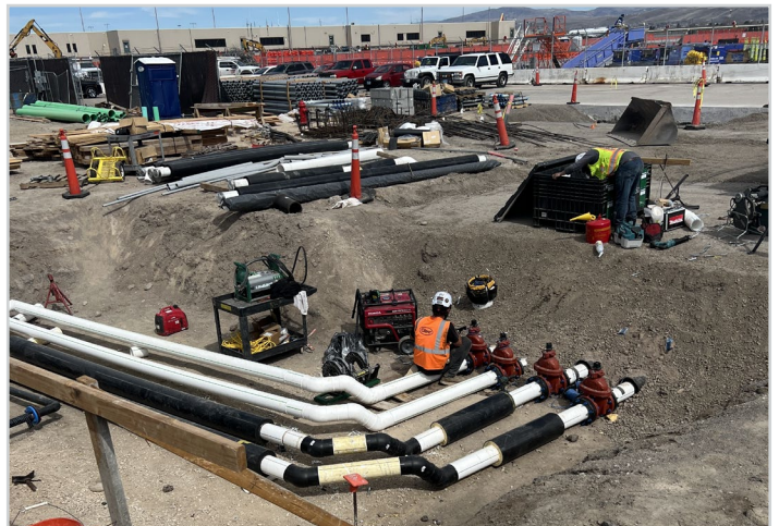
Hot & Cold Water Utility Tie-In
