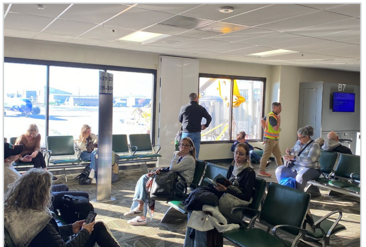
B7 stair demo - door closure
