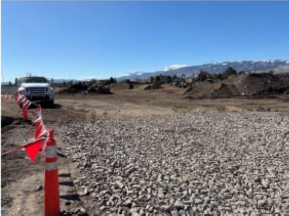
Site Grading Continues
