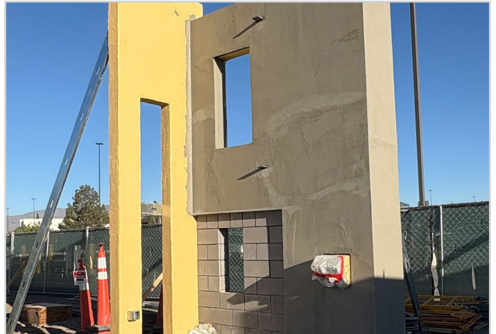
Exterior Finishes Mock-up
