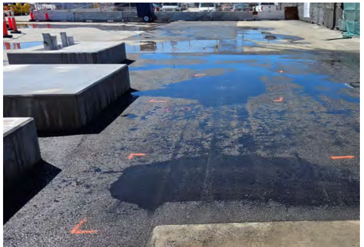
Transformer Pads - New Paving
