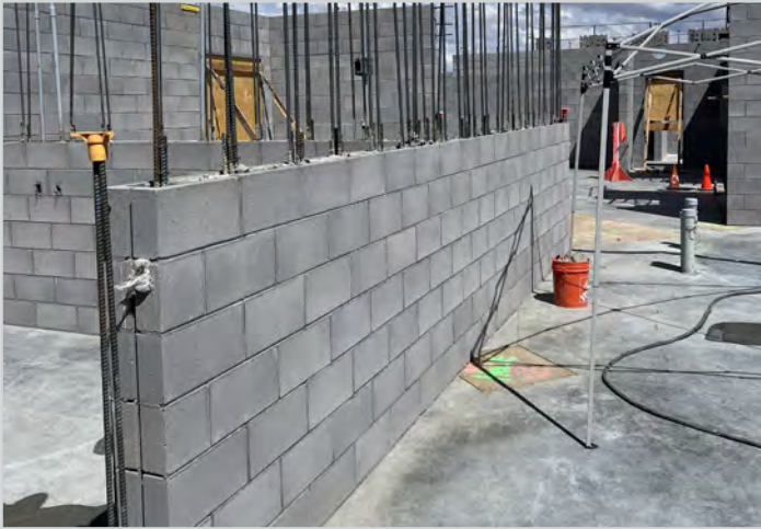
CMU Block Installation
