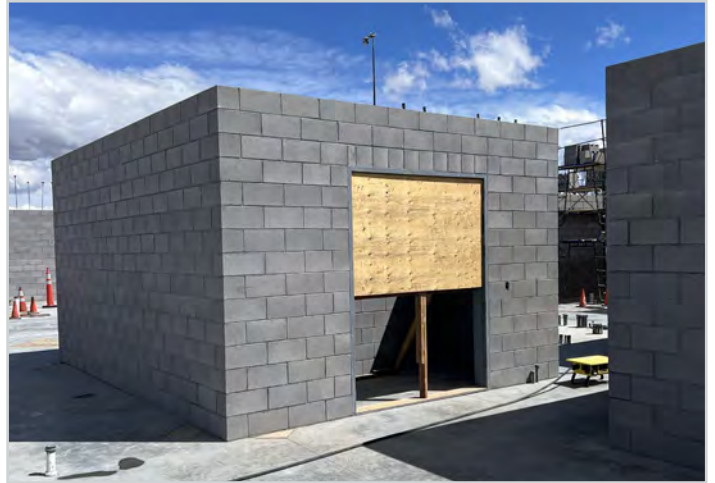
Ammunition Storage Room
