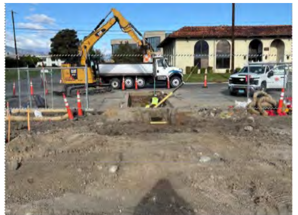
Terminal Way Utility Work
