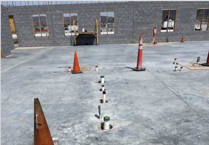
Plumbing Stubs for Police Locker Rooms
