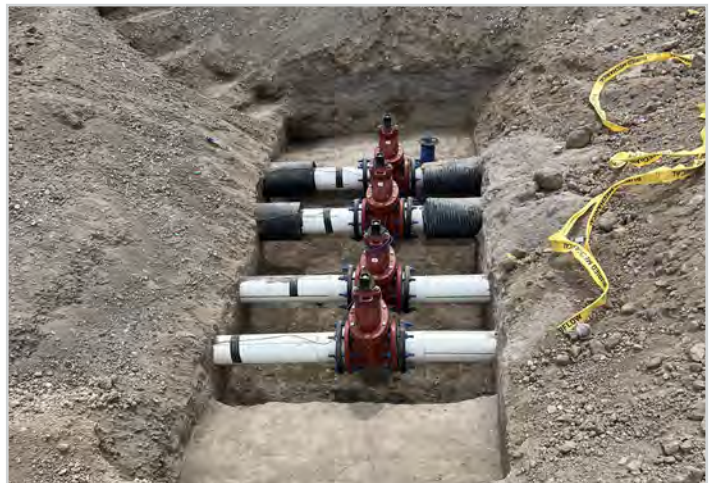
Hot & Cold Water Utility Tie-In
