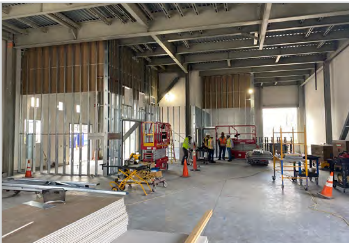
Interior Framing & Drywall
