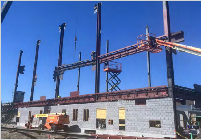
CMU Block & Structural Steel
