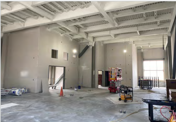
Interior Drywall & Paint
