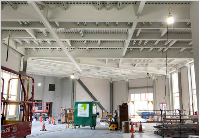
Interior Drywall & Paint
