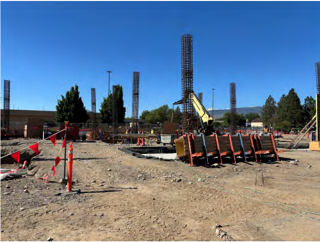
Vertical Columns Started
