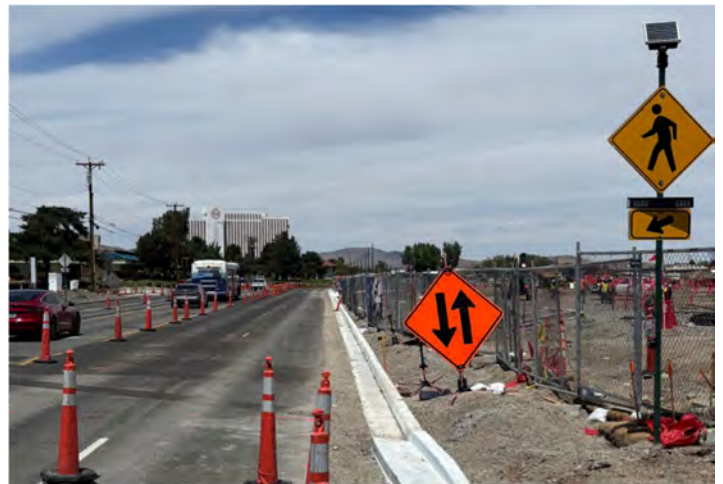
Terminal Way Curb and Gutter
