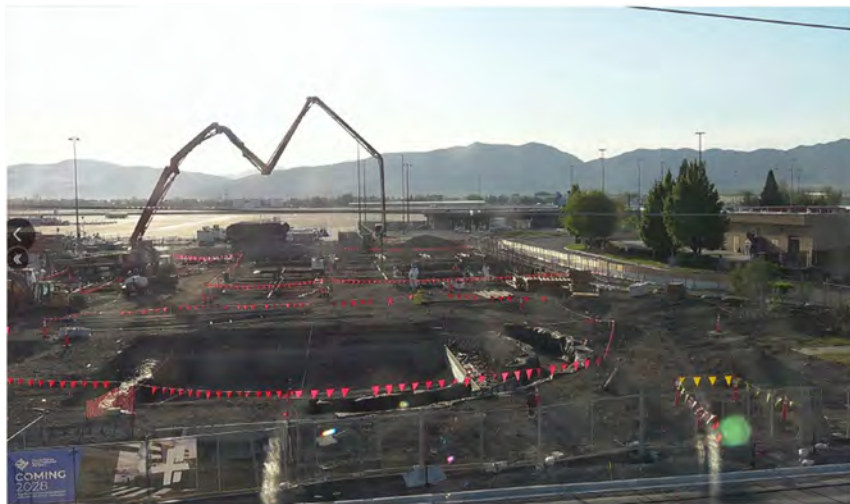
Foundation Placements Started
