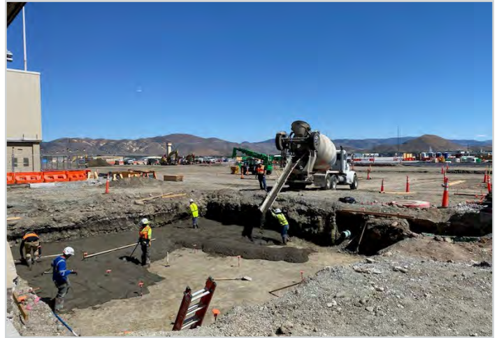
Concourse A - Footing Prep
