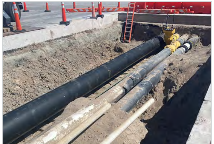
Trench Area 7E - Boring Repair - Casing
