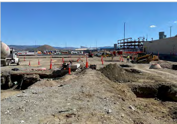
Concourse A - Utility Work
