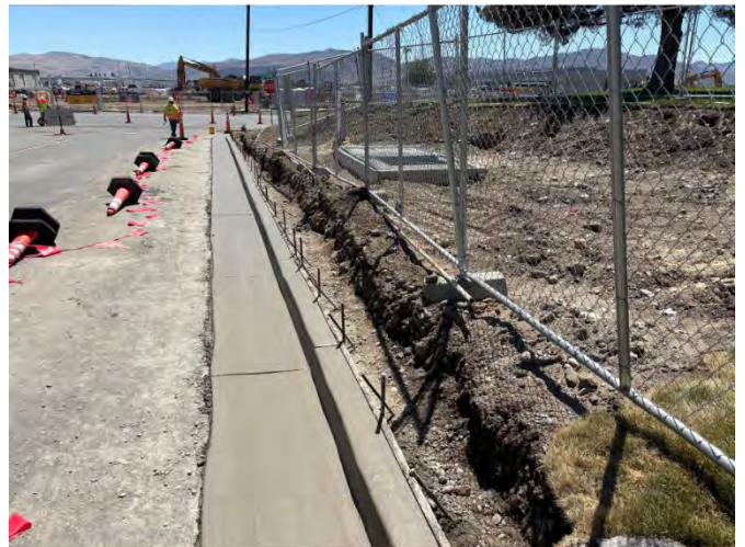
NVE Utilities at Terminal Way
