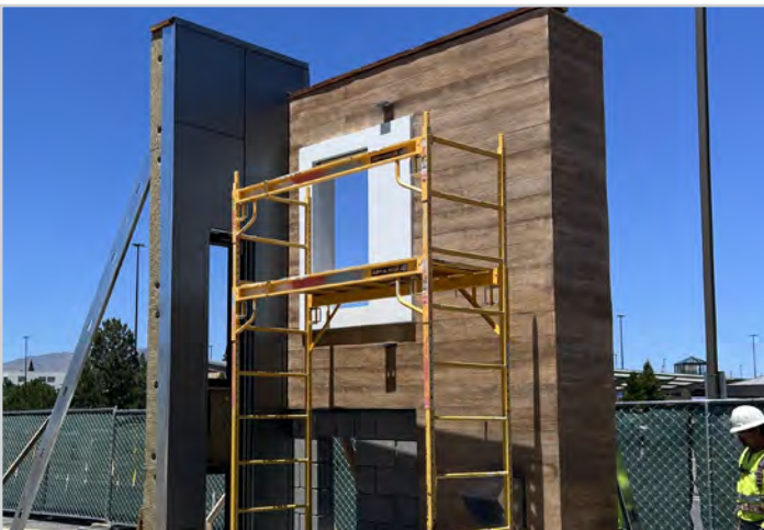
Exterior Finishes Mock-up
