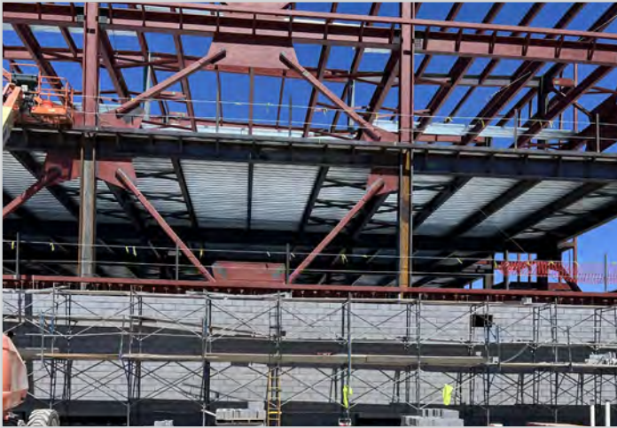
CMU Block & Structural Steel
