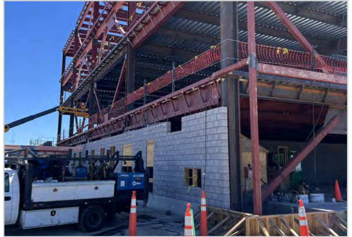
CMU Block & Structural Steel
