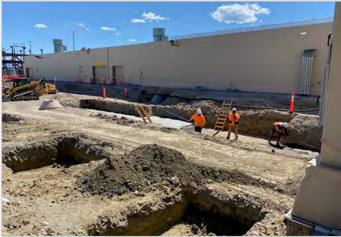
Concourse A - Footing Prep
