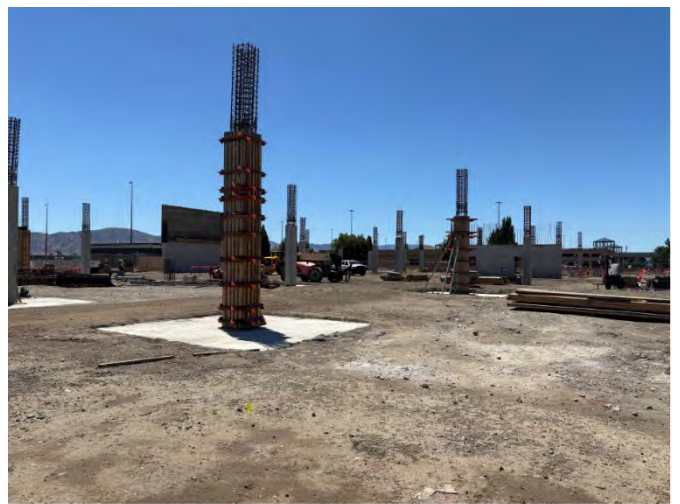
Vertical Columns Continue
