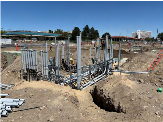
Utility Trenching Continues
