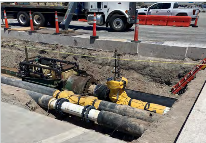
Trench Area 7E - Boring Repair
