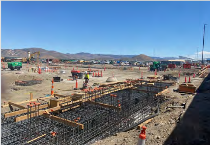
Concourse A - Footing Rebar
