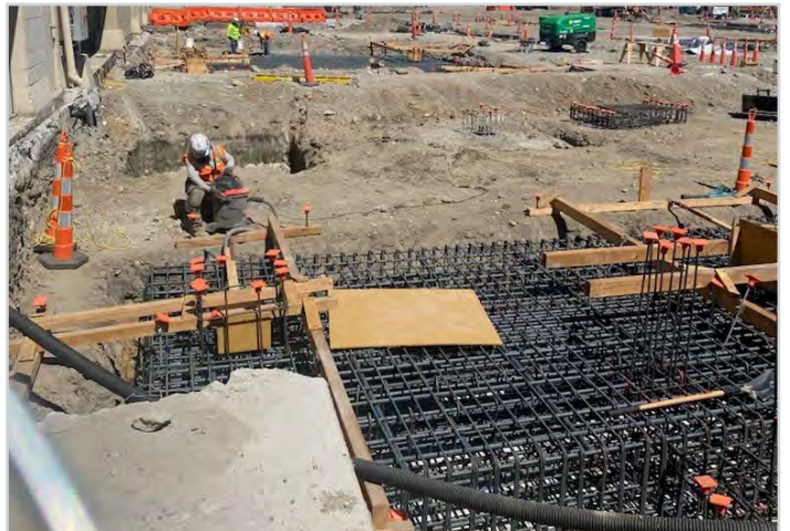
Concourse A - Footing Rebar
