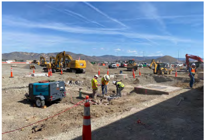
Concourse A - Utility Work
