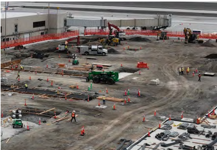
Concourse A - Footing Prep
