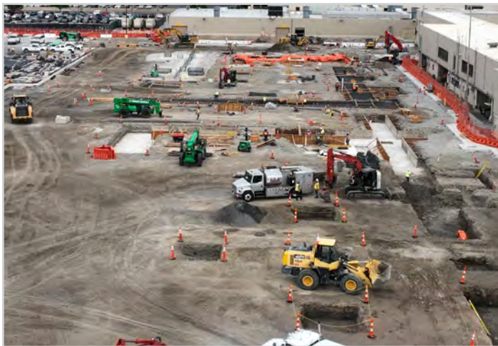
Concourse A - Footing Prep
