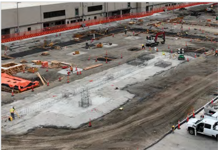
Concourse A - Footing Rebar
