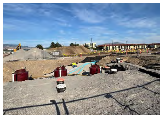
Fuel Tank Installation
