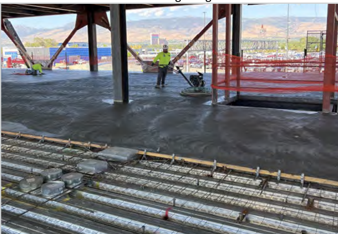
Finishing Concrete on 4th Floor
