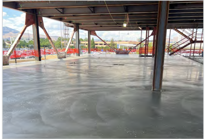
Finishing Concrete on 3rd Floor
