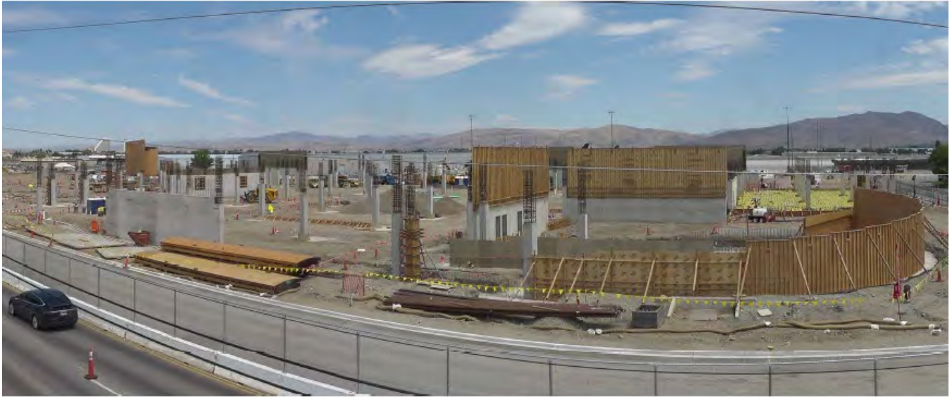
Site Camera Looking NE
