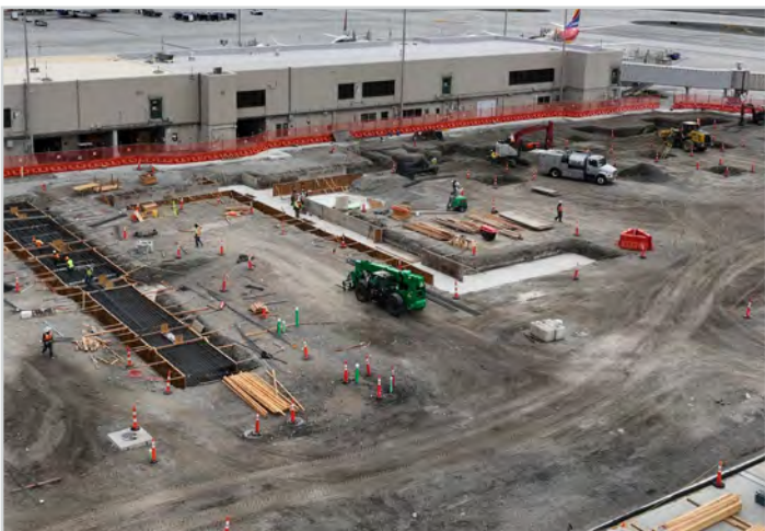
Concourse A - Footing Prep
