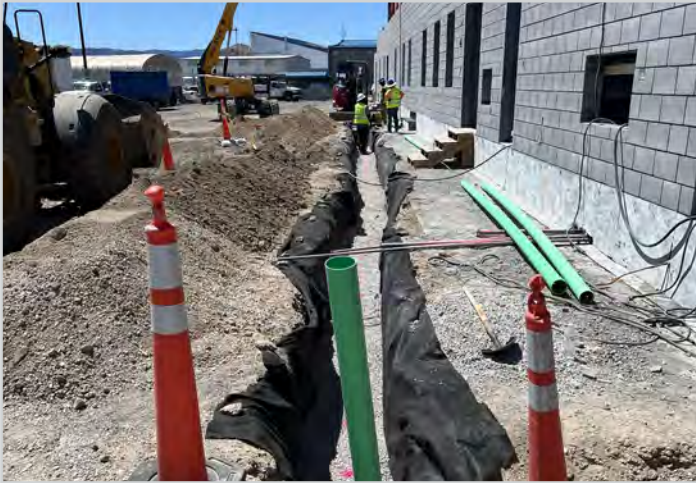
Foundation Drain Installation
