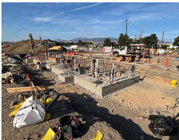
Fuel Station Foundations
