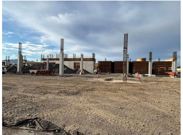
Vertical Columns and Shear Walls
