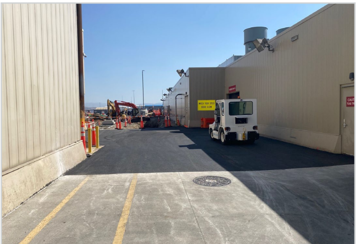
Concourse A - Matrix 2 Paving
