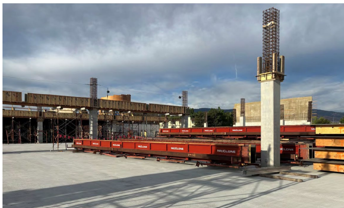
Garage / CSB 2 nd Floor Started
