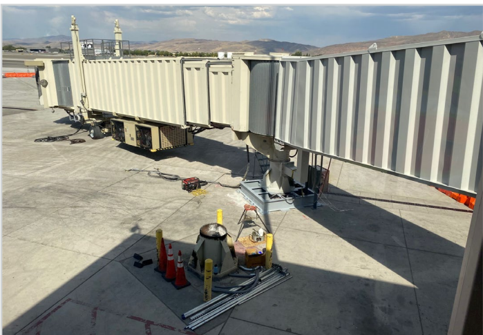
Concourse C - Boarding Bridge Modifications
