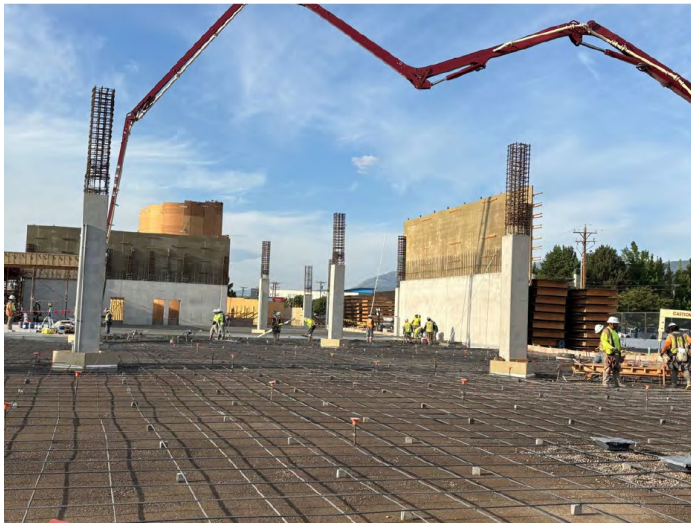
Garage Slab on Grade
