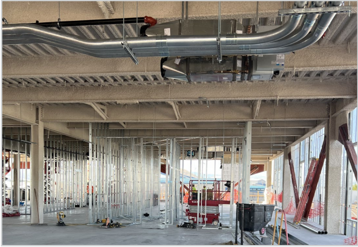
Interior Core Wall Framing - Second Floor
