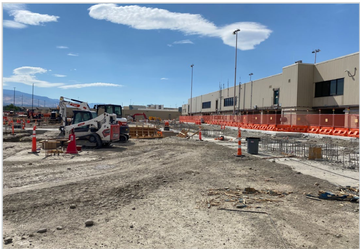
Concourse A - Foundations
