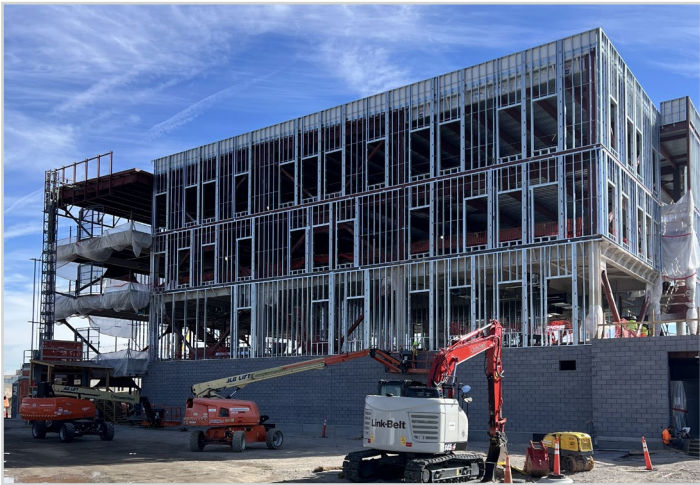
West Elevation - Exterior Framing
