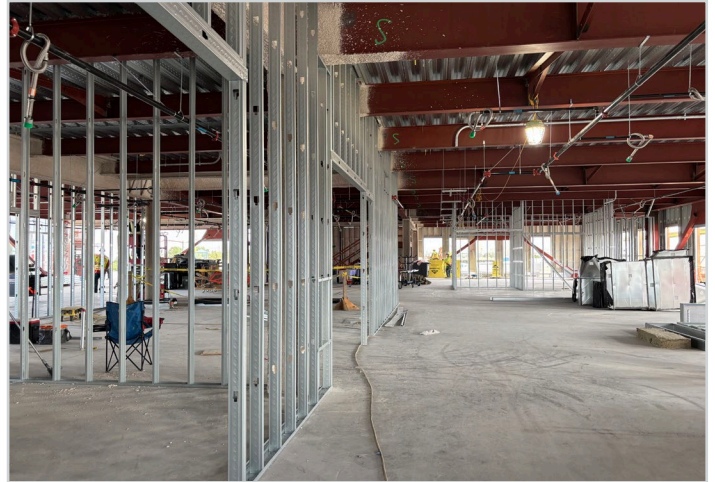
Central Corridor on 3rd Floor
