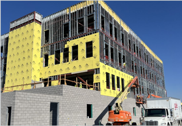
Southeast Corner of the Building
