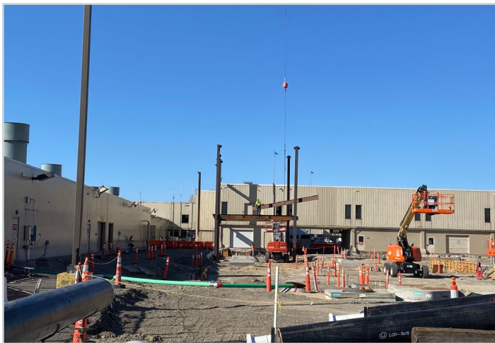
Concourse A - Steel Erection
