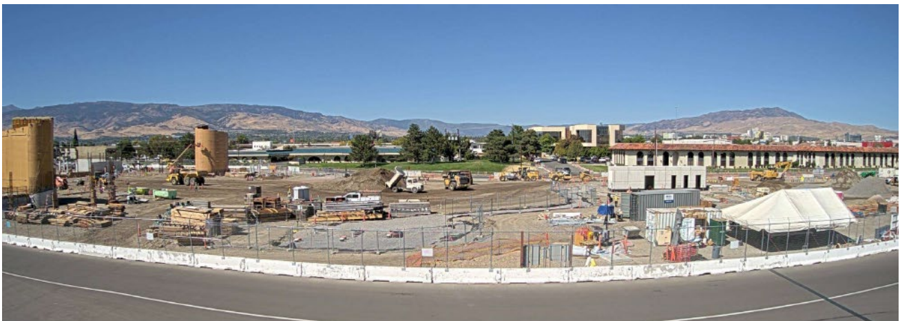
Site Camera at B13
