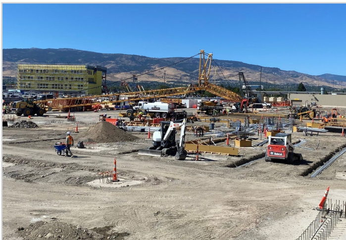
Concourse A - Crane
