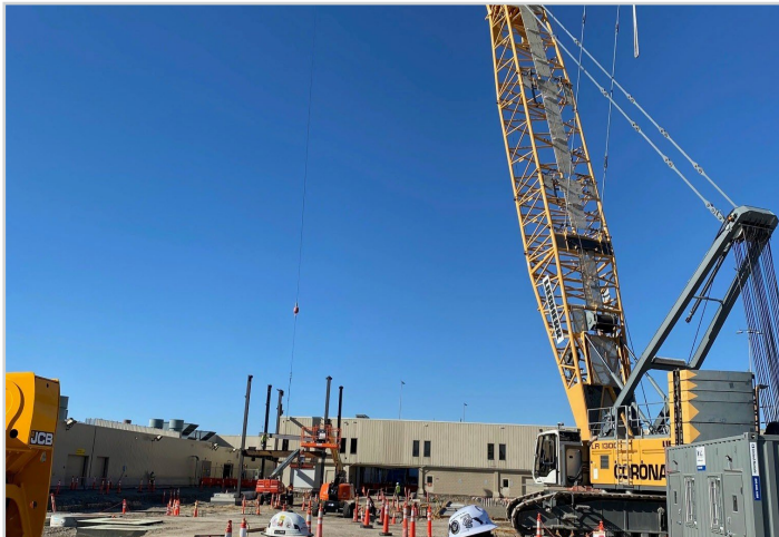
Crane Erecting Steel
