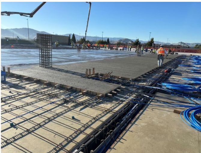
Garage 2 nd Deck Area 2
